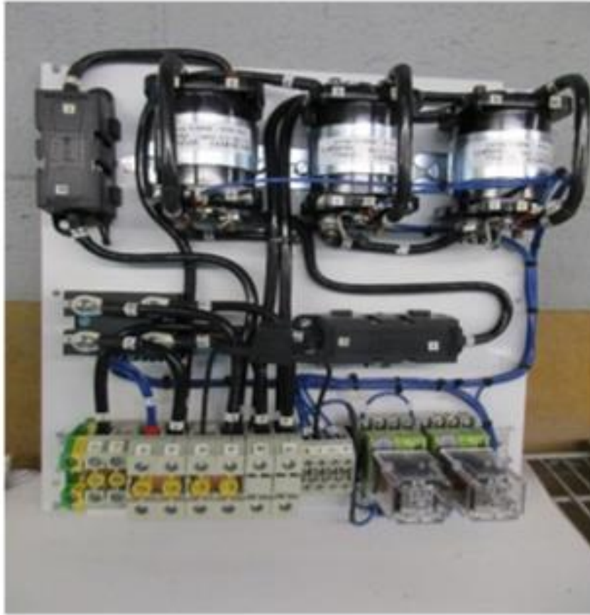
Figure 1. Main Control module for Box
